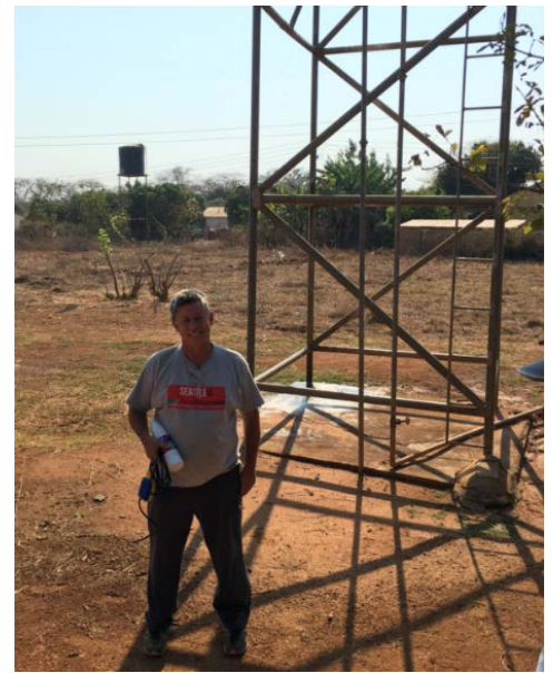
All prepared to replace a water tower float.
