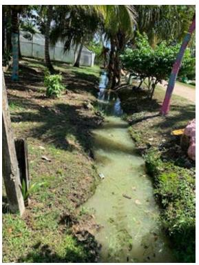
This photo shows the ditch at capacity. The ditch is 3' x 4' x 22'. PWOB is working with SU engineering Professor Mike Marsulak to devise a way to reinforce and stabilize the drainage ditch to prevent continual erosion.
